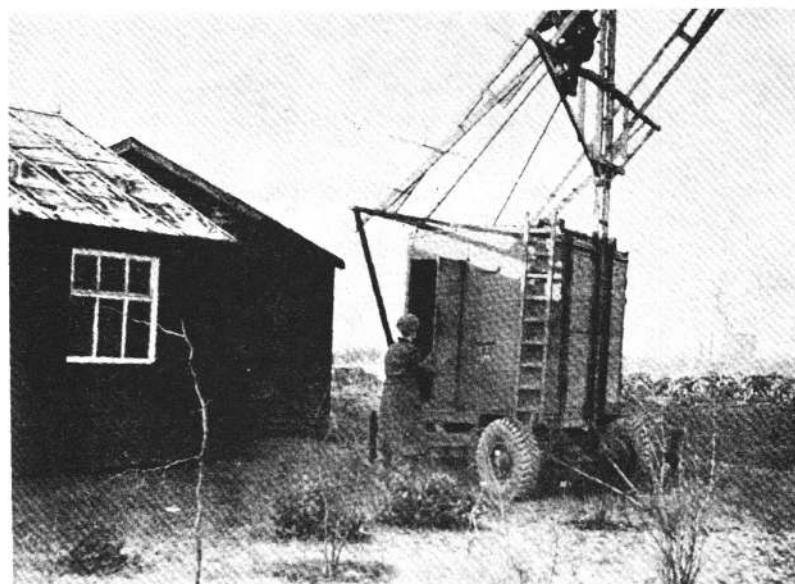
Fig. 5. The first day at Jodrell Bank December 1945. The receiver cabin and Yagi aerial of the 4.2m ex-military radar system, deposited outside huts used by the gardeners of the botanical department.
