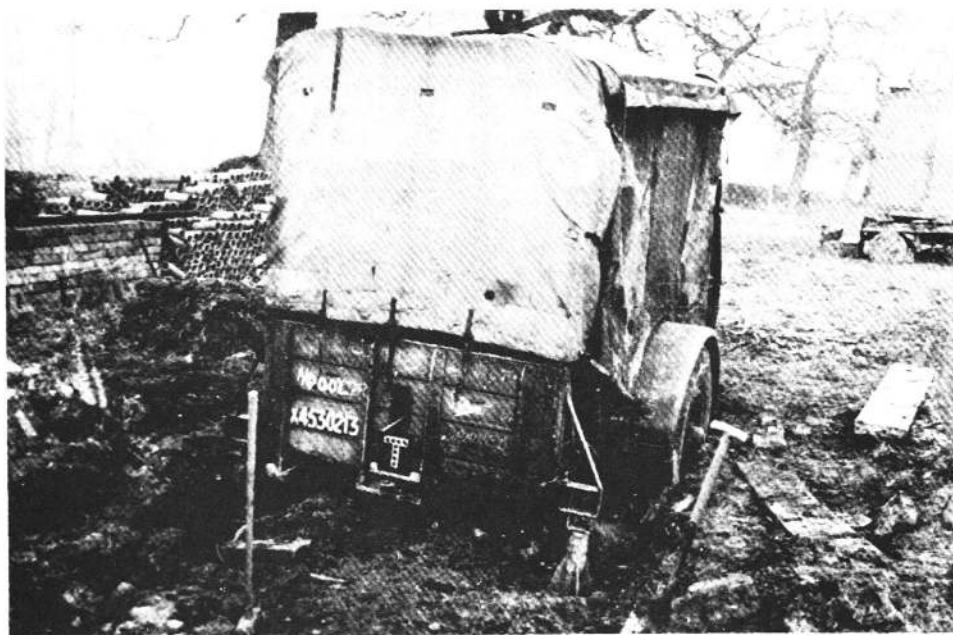
Fig. 6. The first day at Jodrell Bank December 1945. There was no electricity in the vicinity, so power had to be obtained from a mobile diesel generator which is seen here stuck in the mud.
